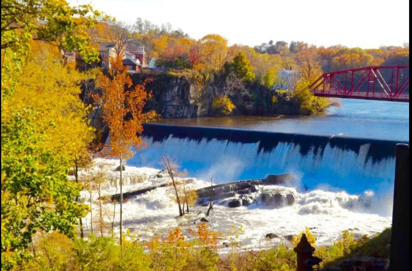
SAUGERTIES DAM, RED BRIDGE
